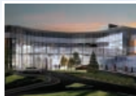
Henderson General Hospital above: New main entrance
